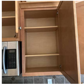
Power Outlets (6/16) 08/02/2024 1:21 PM
