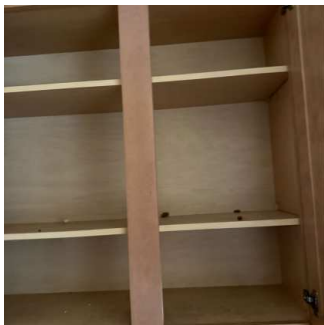
Power Outlets (9/16) 08/02/2024 1:22 PM
