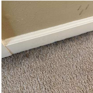
Power Outlets (11/16) 08/02/2024 1:55 PM
