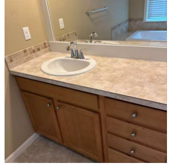
Sink / Faucet (4/16) 08/02/2024 2:06 PM
