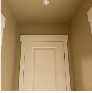
Exhaust Vent (1/16) 08/02/2024 2:05 PM
