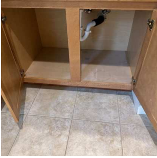
Garbage Disposal (1/16) 08/02/2024 2:06 PM
