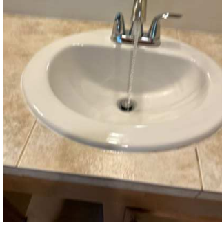
Garbage Disposal (2/16) 08/02/2024 2:06 PM
