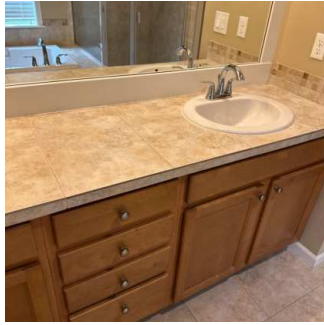
Sink / Faucet (6/16) 08/02/2024 2:06 PM
