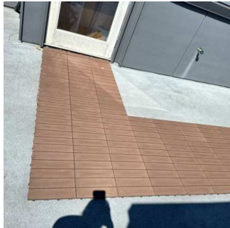
Deck / Patio / Balcony (2/15) 08/01/2024 2:34 PM
