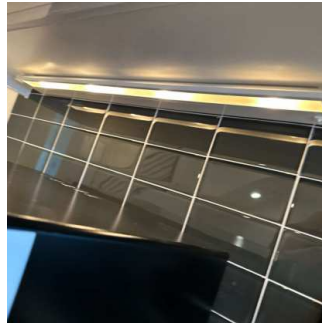
Light fixtures continued (1/16) 08/01/2024 1:54 PM
