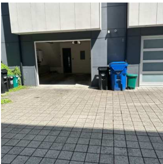
Drive way / carport / parking space (3/3) 08/01/2024 2:39 PM
