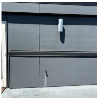
Deck / Patio / Balcony (7/15) 08/01/2024 2:34 PM
