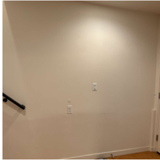
Walls throughout property (2/16) 08/01/2024 1:19 PM
