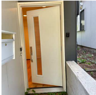
Exterior Doors (2/7) 08/01/2024 1:37 PM
