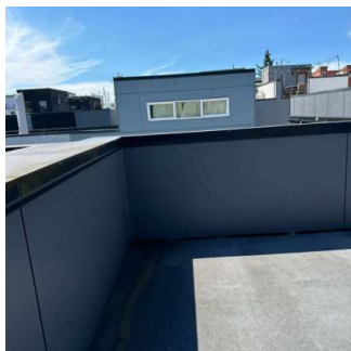
Deck / Patio / Balcony (6/15) 08/01/2024 2:34 PM
