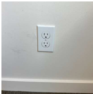
Switches / outlets / wall plates continued (5/16) 08/01/2024 1:30 PM
