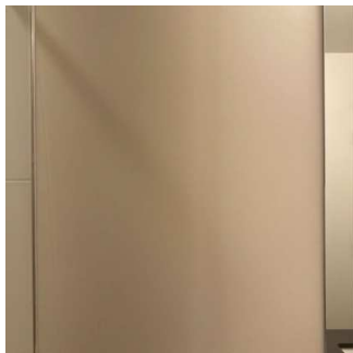
Walls throughout property (14/16) 08/01/2024 1:20 PM
