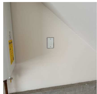
Outlets continued (6/8) 08/01/2024 1:37 PM
