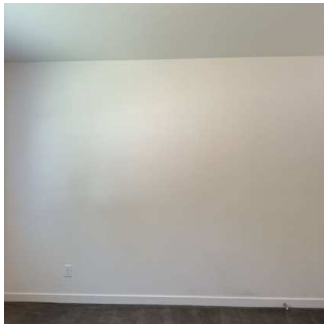
Walls throughout property (9/16) 08/01/2024 1:20 PM
