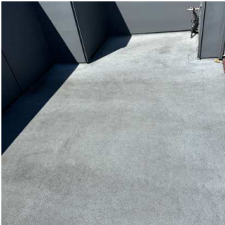
Deck / Patio / Balcony (1/15) 08/01/2024 2:34 PM
