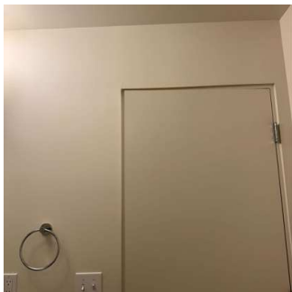
Walls throughout property (13/16) 08/01/2024 1:20 PM
