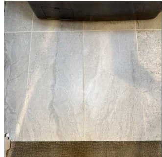
Floors continued (4/8) 08/01/2024 1:46 PM
