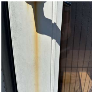
Exterior Doors (6/7) 08/01/2024 1:42 PM
