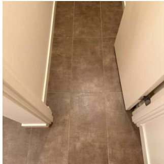
Floors continued (3/8) 08/01/2024 1:46 PM
