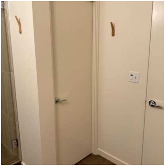
Doors continued (2/7) 08/01/2024 1:41 PM
