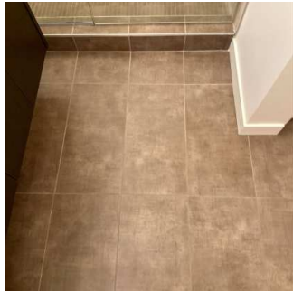
Floors continued (2/8) 08/01/2024 1:46 PM
