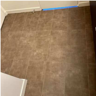
Floors continued (1/8) 08/01/2024 1:46 PM
