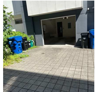
Drive way / carport / parking space (2/3) 08/01/2024 2:39 PM
