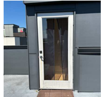
Exterior Doors (4/7) 08/01/2024 1:42 PM
