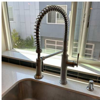
Kitchen Sink & Faucet (2/4) 08/01/2024 2:10 PM
