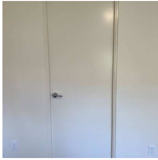
Doors continued (4/7) 08/01/2024 1:41 PM
