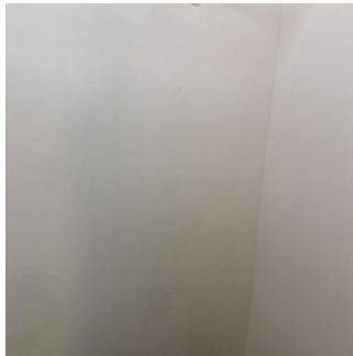
Walls throughout property (11/16) 08/01/2024 1:20 PM
