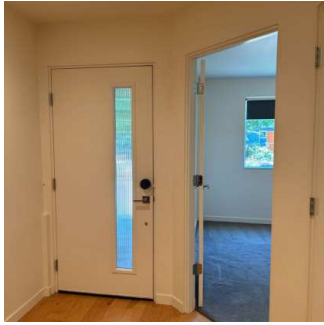
Walls throughout property (1/16) 08/01/2024 1:19 PM
