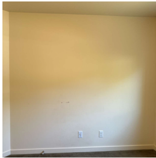
Walls throughout property (7/16) 08/01/2024 1:20 PM
