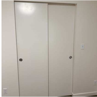
Doors continued (7/7) 08/01/2024 2:26 PM
