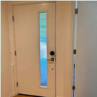
Exterior Doors (1/7) 08/01/2024 1:37 PM
